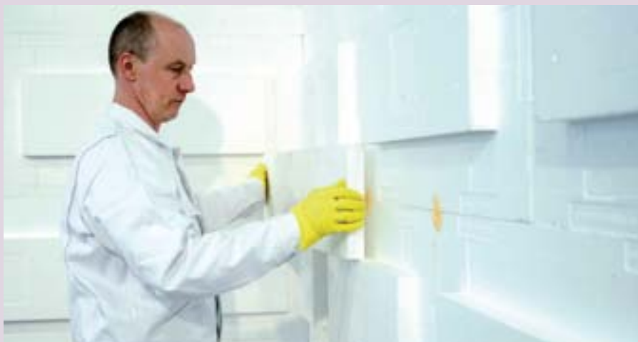
Photo 6 Pose de lockplate.
